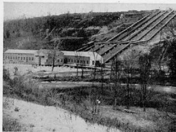
FIG. 2.—PENSTOCKS, POWER HOUSE AND TRANSFORMER HOUSE.
